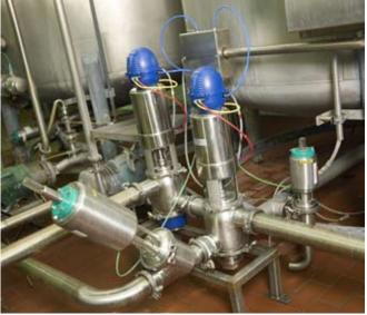
After: new continuous processing line with Unique PMO and PMO *Plus* – *CP* Mixproof valves
